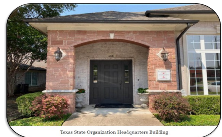
Texas State Organization Headquarters Building
