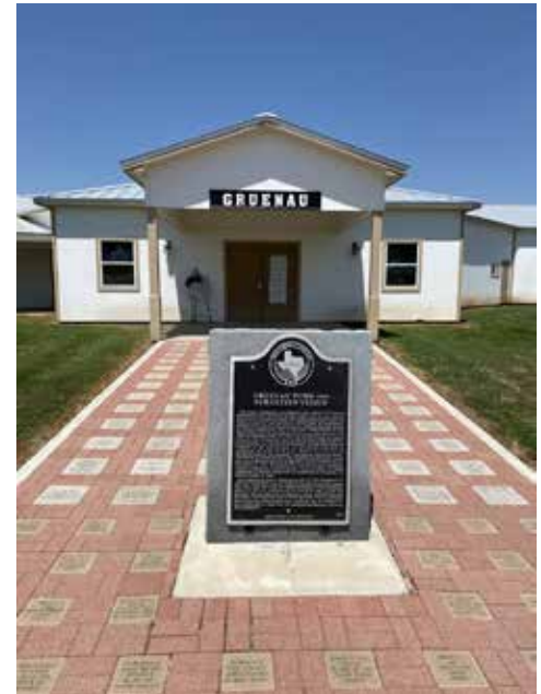
Gruenau Hall, Yorktown, TX
